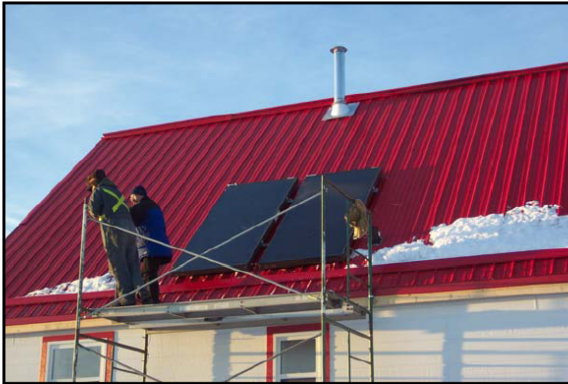
Fig.40 – Scaffolding used for lifting and as work platform
