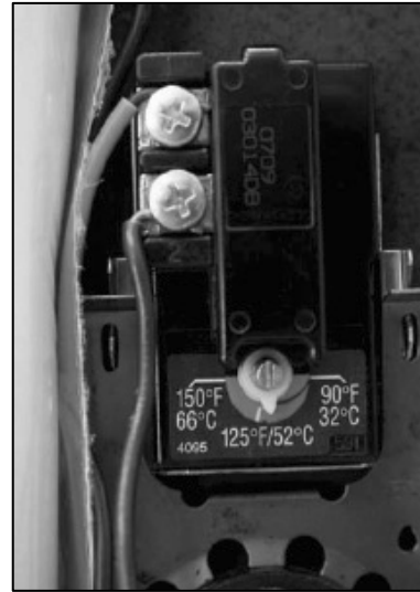
Fig. 4.10.1.5 – Connect red and black wires to Lower thermostat terminals. Set thermostat to 120 °F (50 °C).
