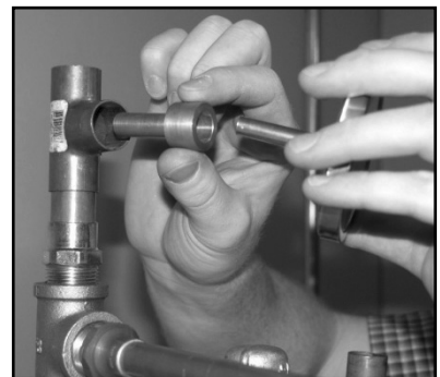
Fig.4.3.3 – Remove thermometer from well
