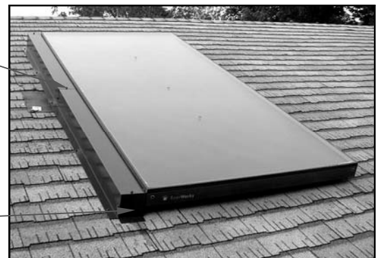
Fig. 7.1.1 – Collector side-flashing. Note roof-penetration boot under side-flashing.
