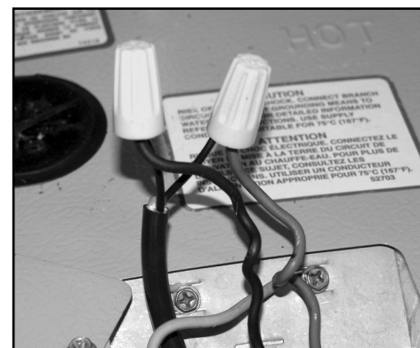
Fig.4.10.1.3 – Connect over-temperature wire to tank wires.
