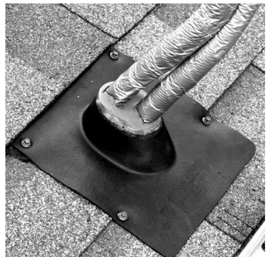
Fig. 5.5.3 – Finished line-set boot flashing.
