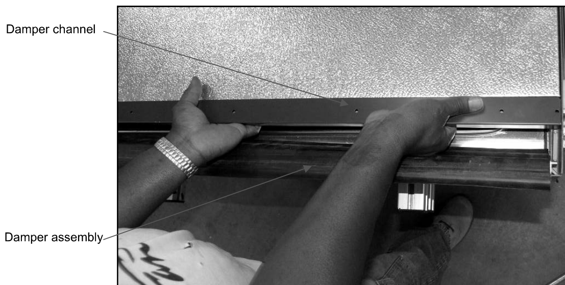
Fig. 6.1.3 – Removing and inserting stagnation-control damper.
