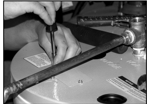
Fig.4.10.1.1 – Remove connection cover plate
