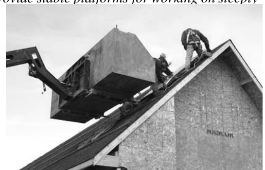
Fig. 6.2.3 – Lifting and securing collectors using forklift boom.
