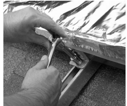
Fig. 6.3.1 – Securing collector with ratchet and extension.
