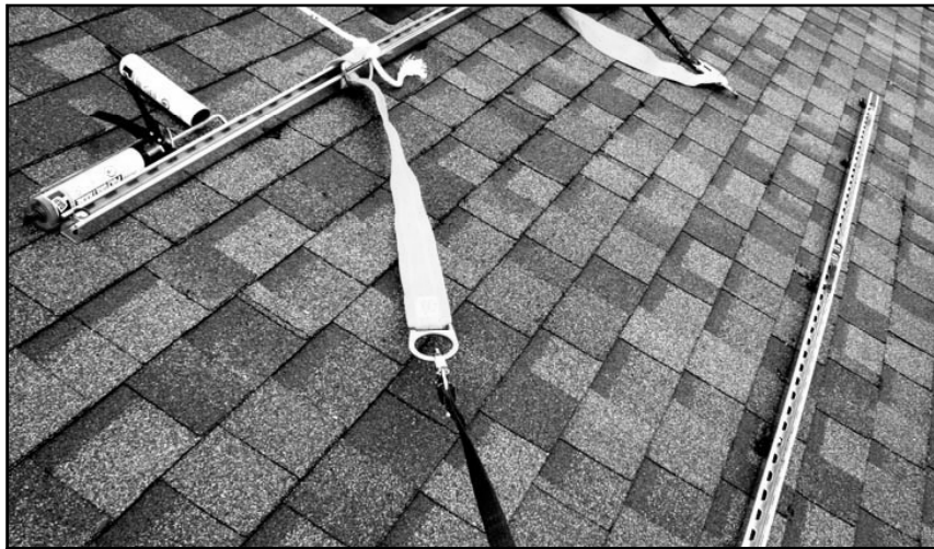
Fig. 5.3.6 – Secured C-channel with safety anchors.
