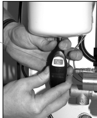
Fig.4.2.2 – Thermistor clamped to corrugated copper pipe close to lower manifold.
