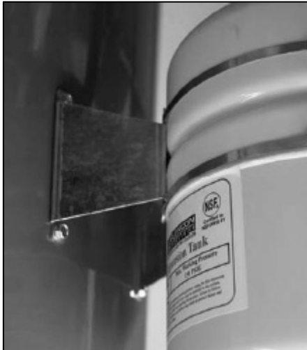
Fig. 4.9.2.1 – Supplemental expansion tank mounted to tank with self-drilling screws.
