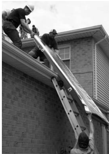
Fig. 6.2.6 – Lifting collector to roof using ladder and lines.
