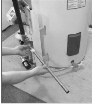
Fig. 4.5.1 – Fabrication of heat trap using a flexible corrugated pipe to cold mains inlet. Using two hands bend pipe down and back (not included).
