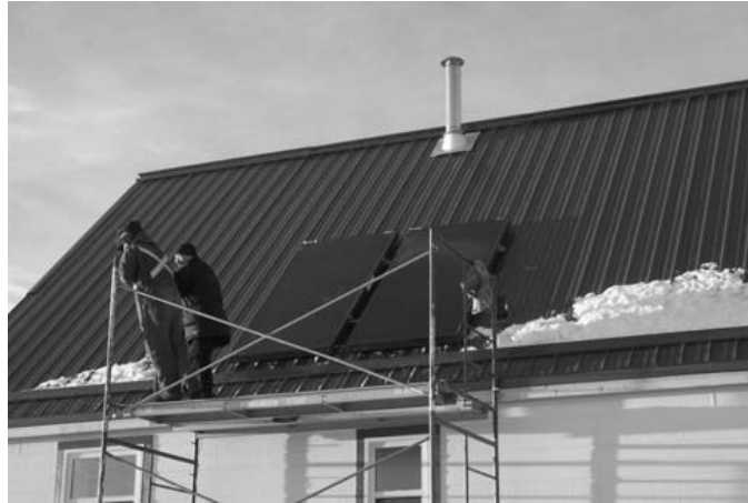
Fig. 6.2.4 – Scaffolding used for lifting and as work platform.
