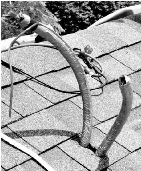
Fig. 5.5.1 – Line-set and control wire protected with tape.
