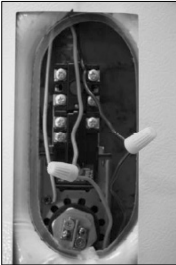
Fig. 4.10.1.4 – Connect wires to bypass upper thermostat.
