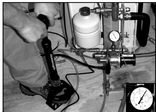
Fig.5.1.2 – Leak-test: pressurize appliance to 40 psi and wait 30 minutes.
