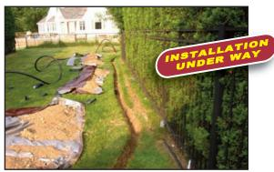
Shallow trenching for pool feeder pipes.
