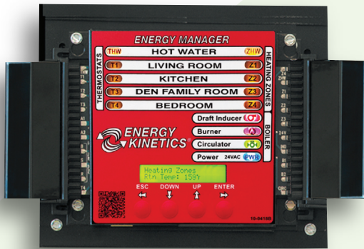
Lights indicate hot water production.
