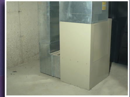
Hydro-air and heat pump backup
